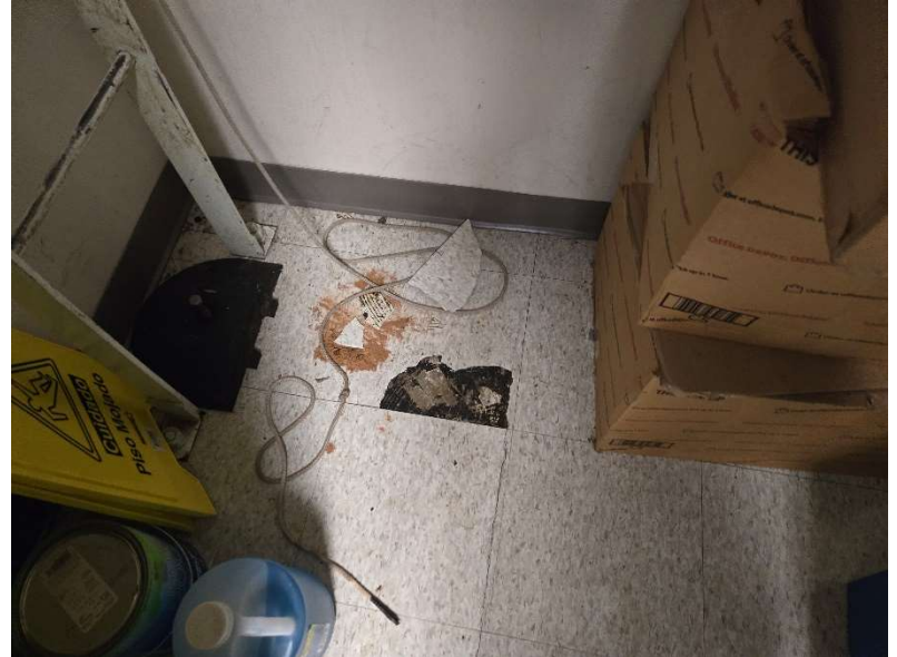
Photo: Black mastic under tile in Room 2.
