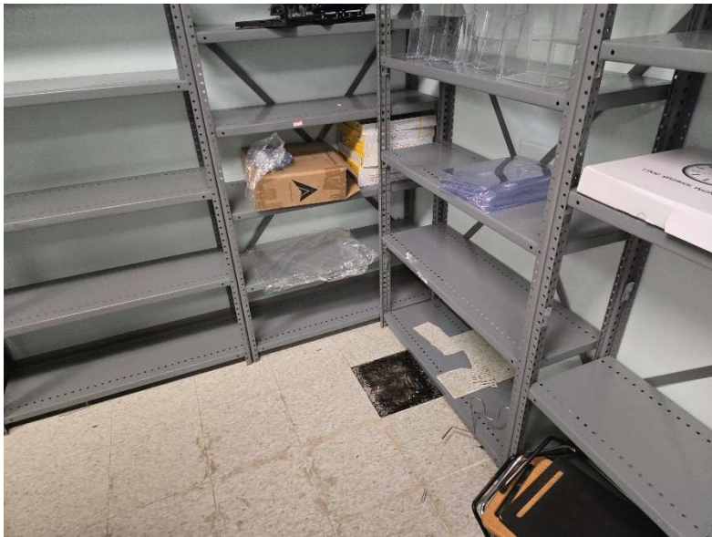
Photo: Black mastic under tile in Room 3.
