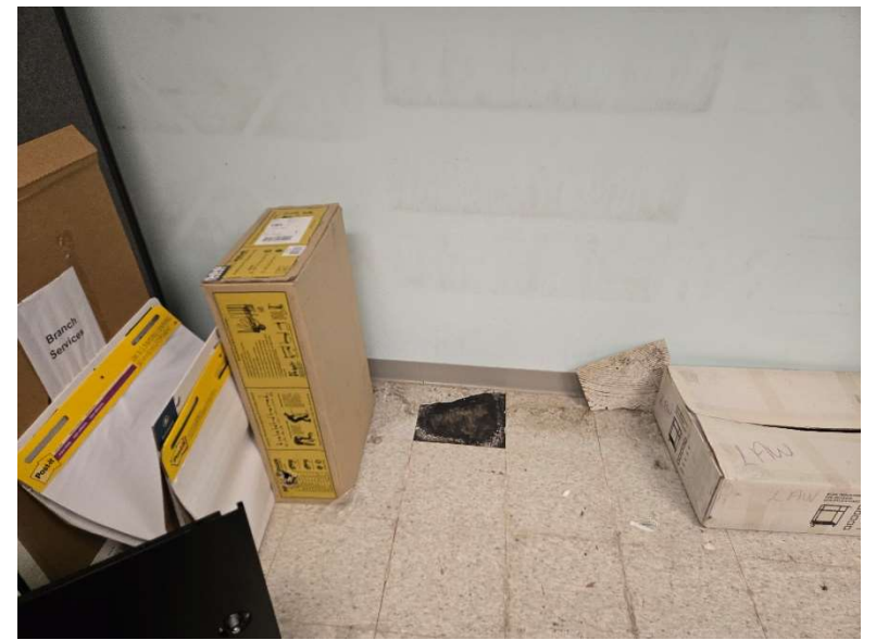
Photo: Black mastic under tile in Room 3.
