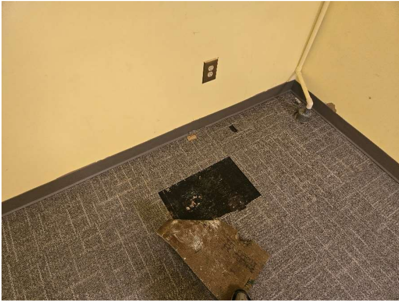
Photo: Black mastic under carpet tile in Room 1.
